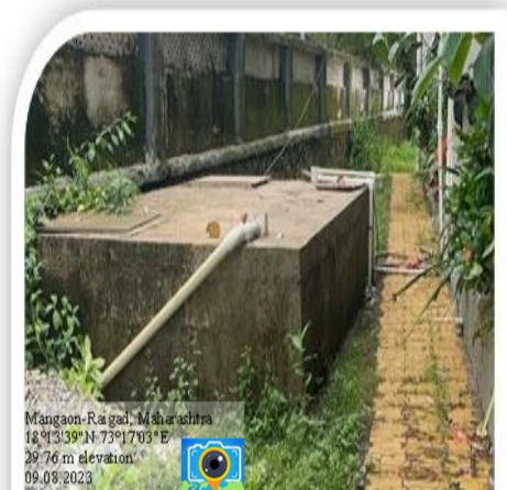
Underground water tanks
