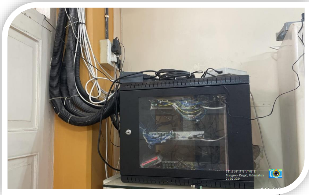
Repairing and maintenance
